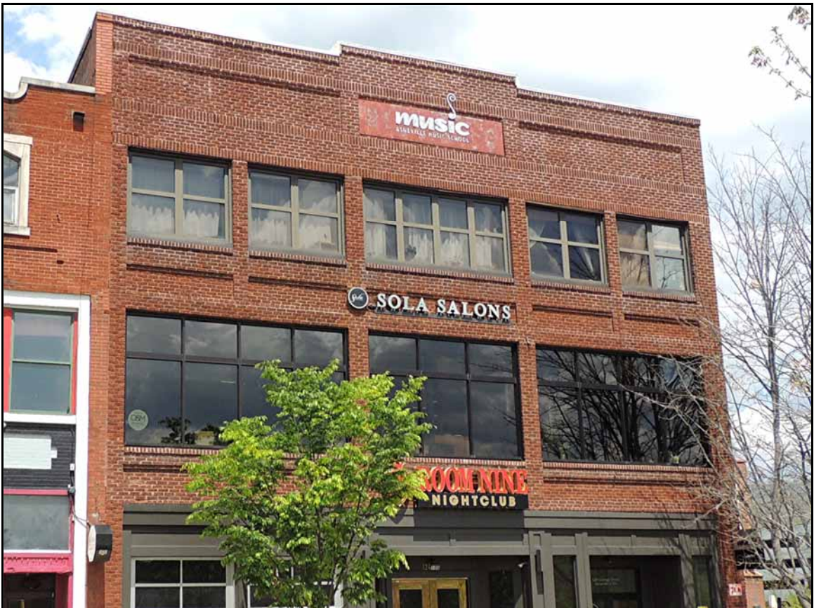
The brick work on this building face has many indented layers.
