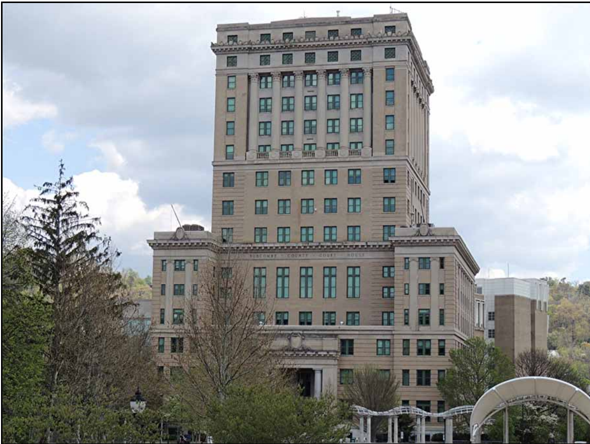
This massive stone structure is a bit out of place in Asheville. This is the kind of structure one might see in New York city.
