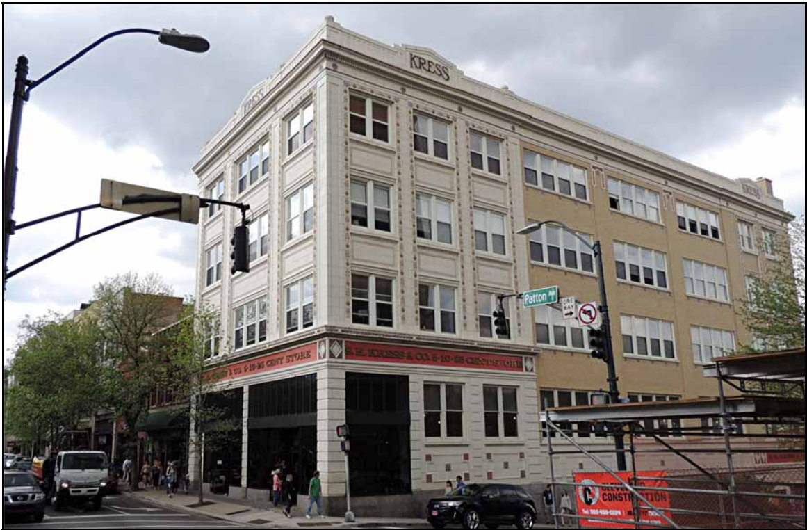
The yellow brick area of this building was added at a later date and while the builders tried to match the stone top they got close, but it is slightly off.
