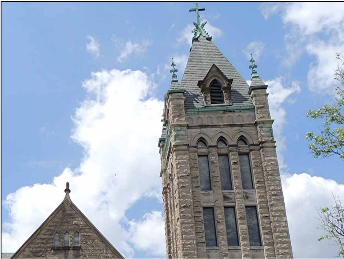
Note the green staining on the stone bleeding off the copper. The green color is almost identical to the tarnishing of the copper at the Biltmore house.
