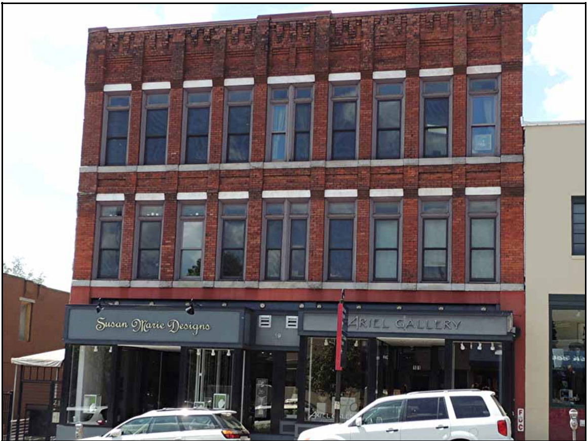
The brick work at the upper area of this building is extensive, however much of it is hard to see at first glance due to the staining.
