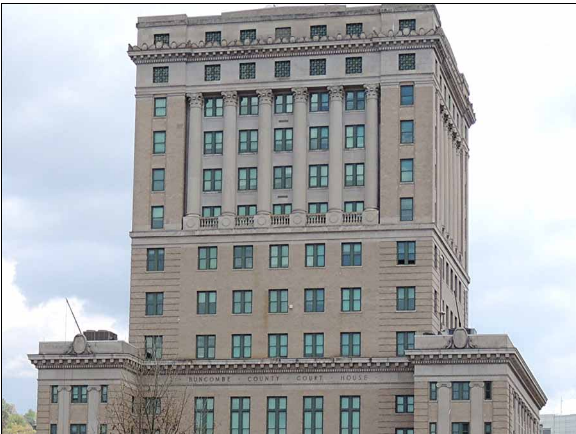
A closer view shows the stone carvings at the top of the columns, the ornamental area at the top and the stone railings at the base of the columns.
