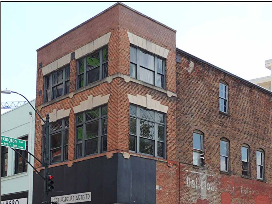
The brick color and lack of stone work above the windows indicates that the back half of the building was added at a later date.
