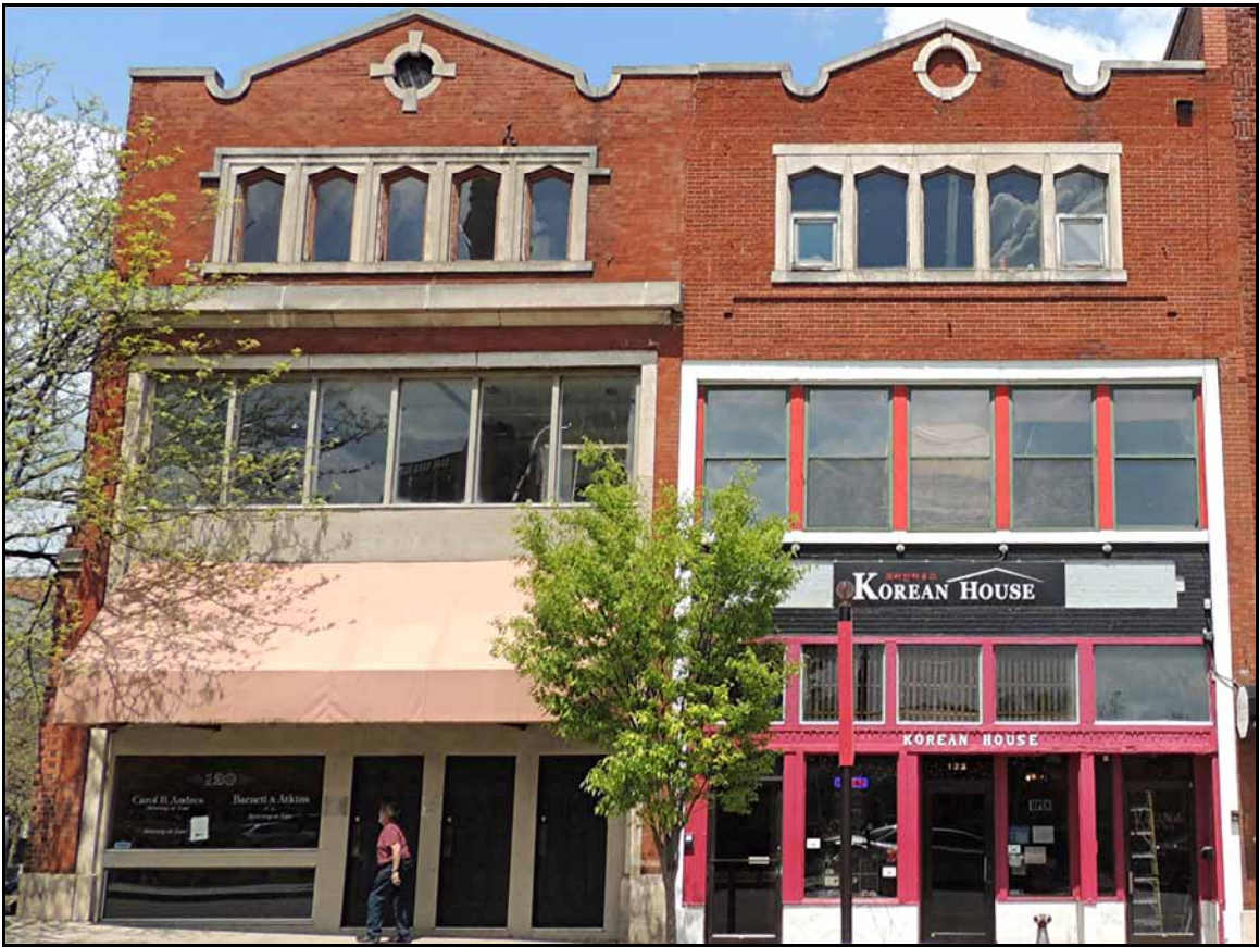
The stone work around the upper windows is interesting. Also note the stone caps at the top of the brick.
