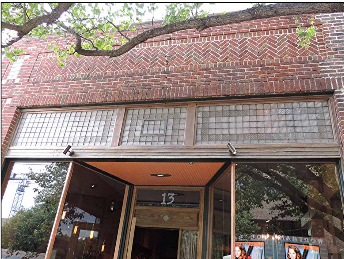
Another example of brick work however this building front also incorporated glass blocks.
