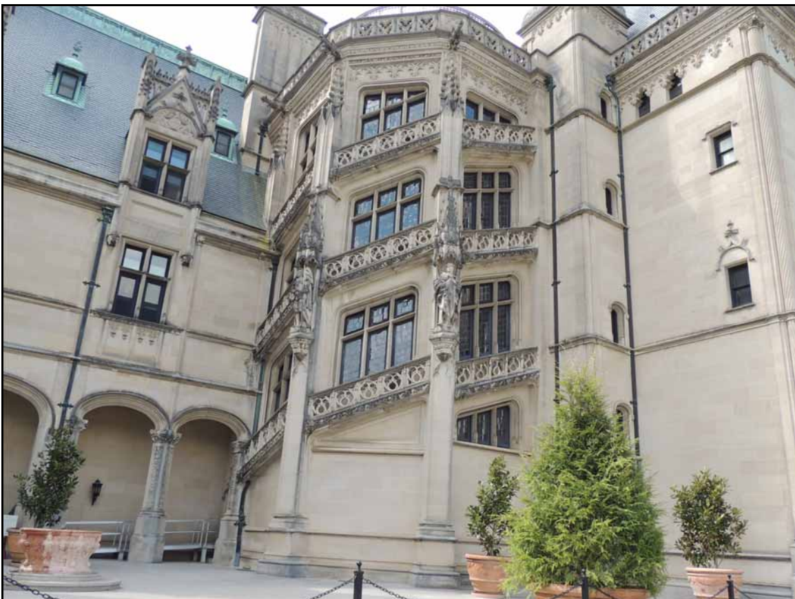
There are a lot of carvings in the stone. Note how the mold and grime is on the tops and bottoms of the carvings.
